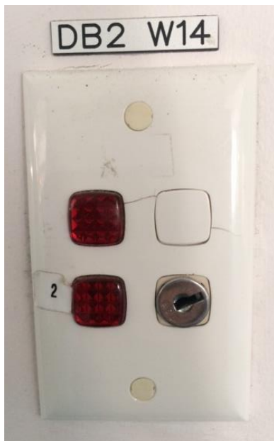
Lights are off = the doors are unlocked
