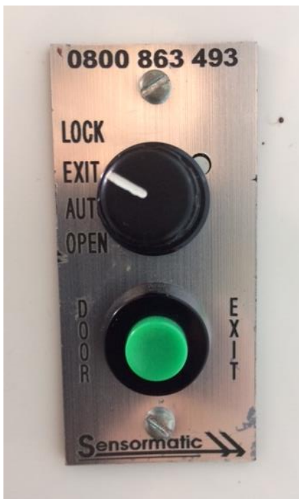
Inner door controls. Turn dial to 'EXIT'.
