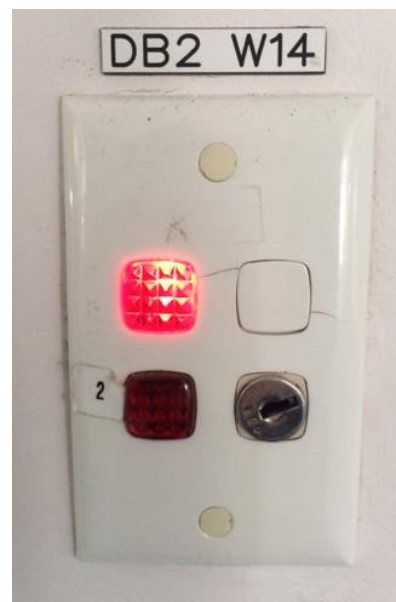
Light is on = doors are locked (only one panel light needs to be on)
